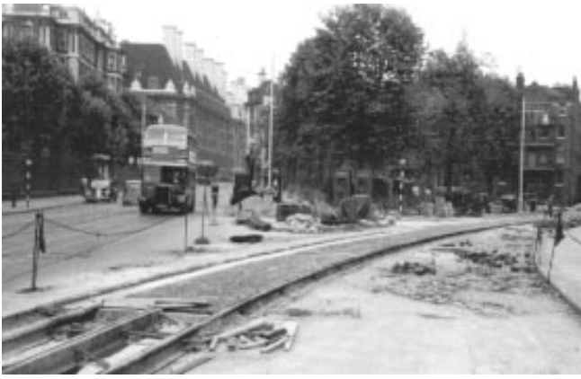
A nearly complete section of track at the end of one of the diversions. (detours) The area between the tracks has been paved up to the point where access is still needed to connect up the current conductors. (live rails) The long yoke holds the running rails and the conduit beams and the short yoke holds only the conduit. No power rails have been laid in yet: they will be held up by insulators attached to the lower flange of each side beam of the conduit.
