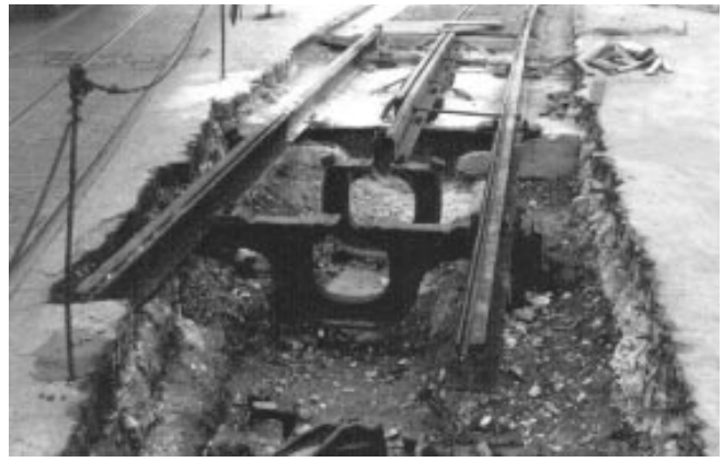
A nearly complete section of track at the end of one of the diversions. (detours) The area between the tracks has been paved up to the point where access is still needed to connect up the current conductors. (live rails) The long yoke holds the running rails and the conduit beams and the short yoke holds only the conduit. No power rails have been laid in yet: they will be held up by insulators attached to the lower flange of each side beam of the conduit.
