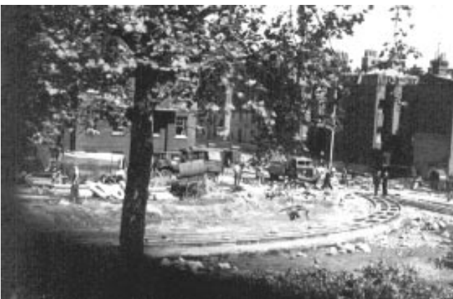
Construction next to a tree.
