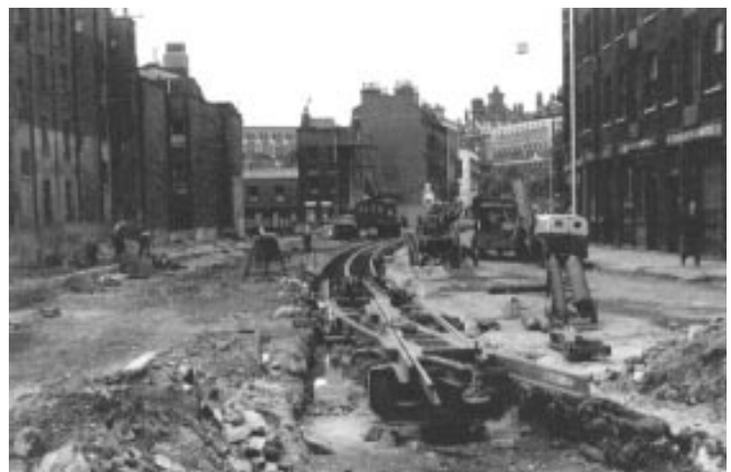
Turnout tracks are supported on concrete pillars.
