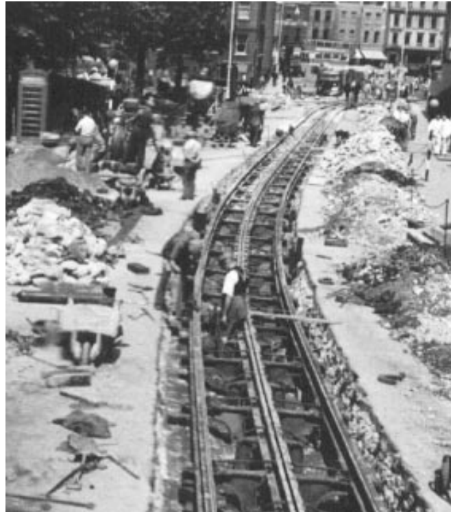
A nearly complete section of track at the end of one of the diversions. (detours) The area between the tracks has been paved up to the point where access is still needed to connect up the current conductors. (live rails) The long yoke holds the running rails and the conduit beams and the short yoke holds only the conduit. No power rails have been laid in yet: they will be held up by insulators attached to the lower flange of each side beam of the conduit.
